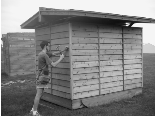
Figure 2. Wearable computers allow construction personnel access to project information at the point of work on site; here the computer is tucked into the constructor's nail pouch.
